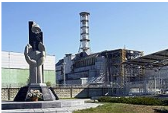
The concrete sarcophagus around the destroyed reactor, which was quickly erected after the accident, started to fail. Below are hundreds of tons of molten nuclear fuel and huge amounts of radioactive dust.
