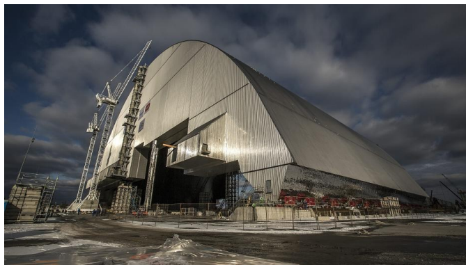
New protective cover for nuclear power ruin. (Photo: dpa, EPA / EBRD Photostream). It is supposed prevent radioactivity leakage for 100 years.
